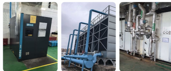
On-site Image of Energy-saving Technological Transformation Projects
